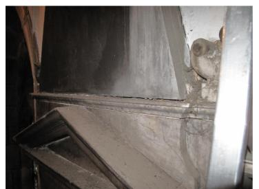
The western side of the obelisk is lifting due to the jacking from an internal ferrous fixing.
