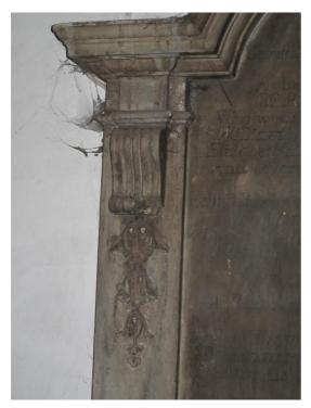
Detail of the east side cornice bracket showing a detail of the stains caused by water running across the surface – as suggested above probably as a consequence of the roof leaking at some point?
