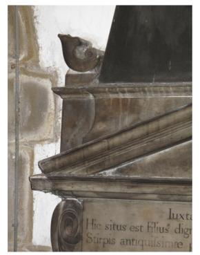
Detail of the east side horn with evidence of additional water runs across the surface at this point.
