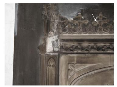
Detail of the missing eastern pilaster capital and damage to the crocket as indicated by the white arrow.
