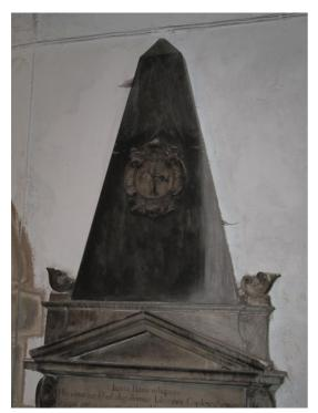
Detail of the upper sections of the monument showing clearly the impact of the water running across the surface.
