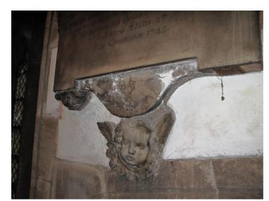
General view of the underside area adjacent to the east corbel showing where the latter is missing.
